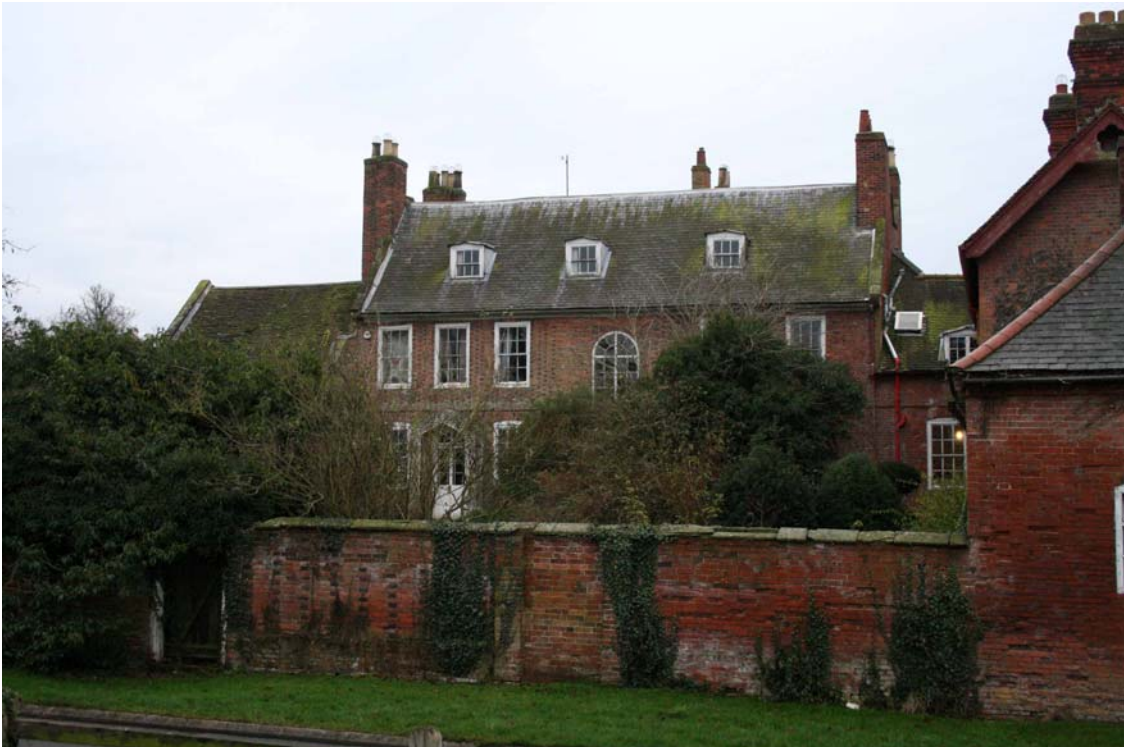
Fig.2 - Cotesbach – Cotesbach Hall (from raised churchyard) - SP 53900 82411 \pm 5 m, bearing 148° OAA 6320]
